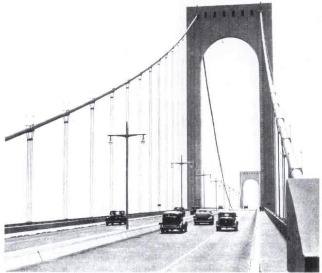
Bronx-Whitestone Bridge; NY, NY, circa 1937. Original deck was 212,400 square feet of 4 1/4" I-Beam Lok that is still in service today.
