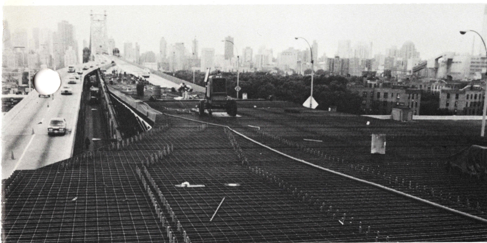
Rehabilitation of Queensboro Bridge, New York City, N.Y.
