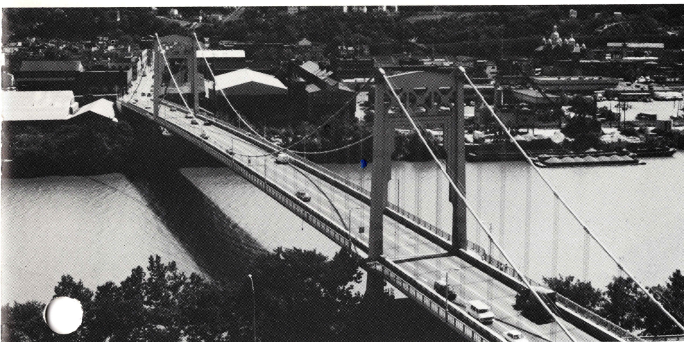
Tenth Street Bridge, Pittsburgh, PA, 3" Full Depth Grid Installed 1932
