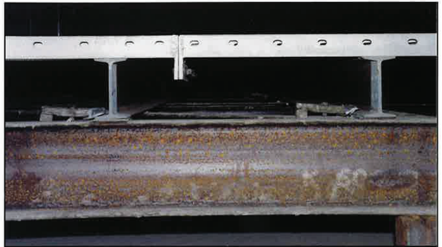
Grid end plates were bolted at longitudinal joint, between stringer supports.
