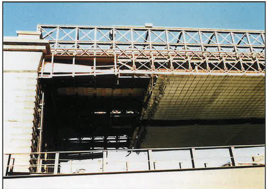
Below-deck work platforms important to timely completion of project.
