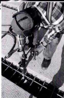
Top Photo: Overnight Deck Replacement Above Left: Shear Stud Placement Above Right: Built-in Leveling Bolt and Transverse Shear Key Below Left, Bottom: Grid Panel Positioning Below Left, Upper: Concrete Placement - Cast-in-Place Deck
