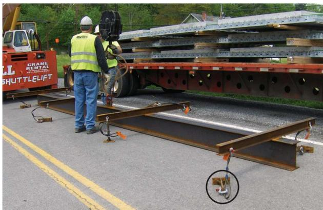
WT shape lifting device (circled).
