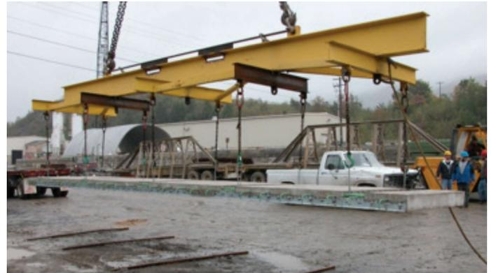
*Left and Above: Examples of Rigid Lifting Frames.*
