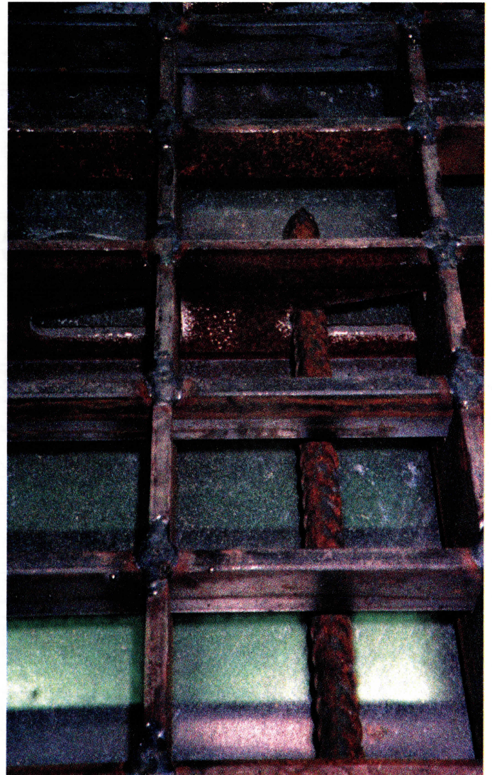
Photo 2 Splice Rebar May be Inserted Through Grid Cross-bar slot, or Through Separate Opening at Option of Grid Manufacturer.
