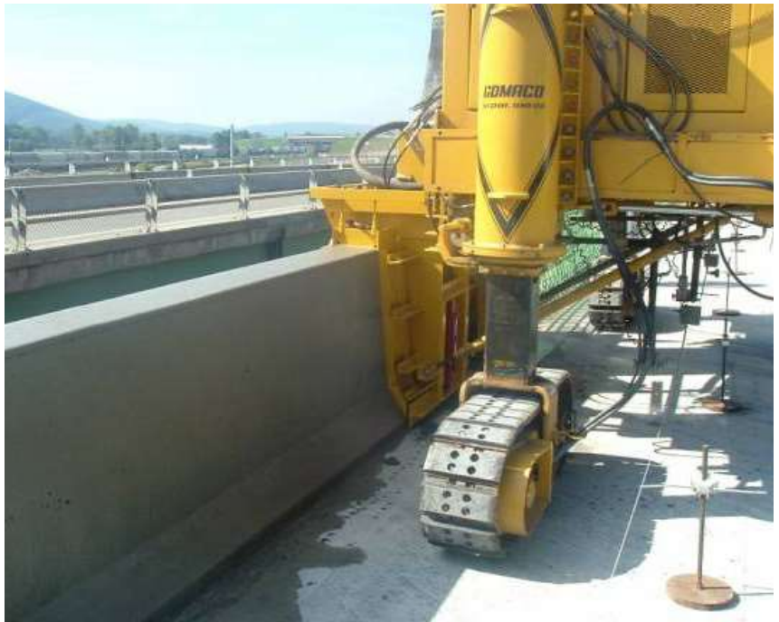
Concrete barrier being placed during slip-form operation.
