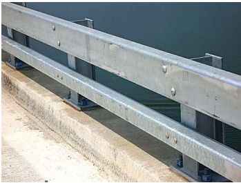
Combination concrete parapet and metal railing.
