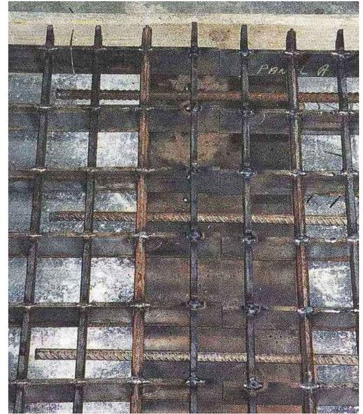
Grid with rebar splice prior to concrete
