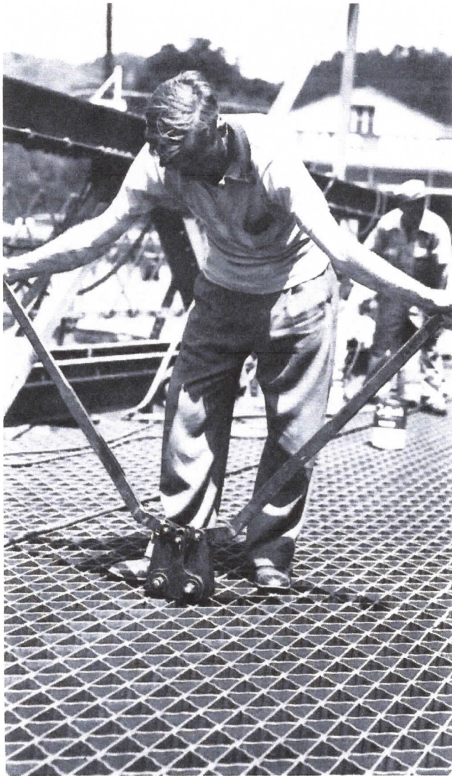
Riveting the splices.
