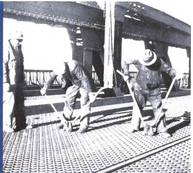
Riveting Splices
