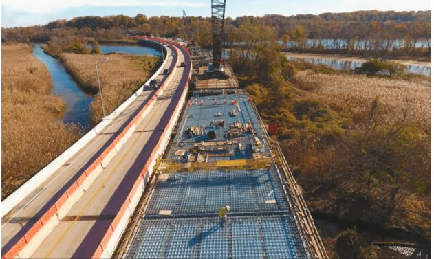
Panels were put in place to prepare for cast-in-place pour
