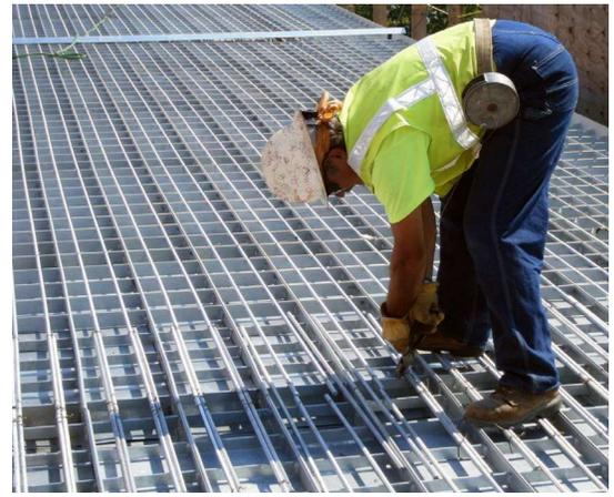
*Installation of Galvanized Grid and Rebar*
