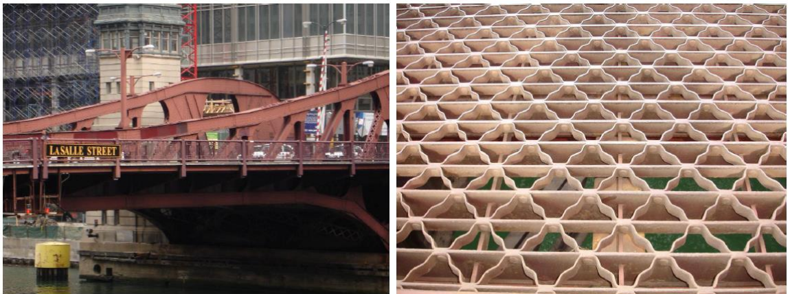
Figure 1.2 - The LaSalle Street Bridge in Chicago installed with riveted deck in 1971
