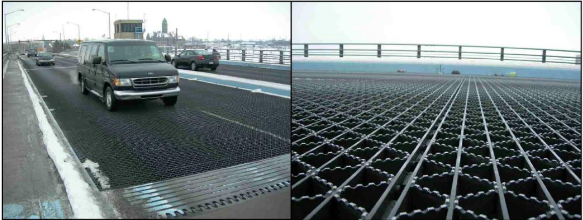
Figure 1.1 - Veterans Memorial Bridge, Bay City with Heavy duty riveted gratings
