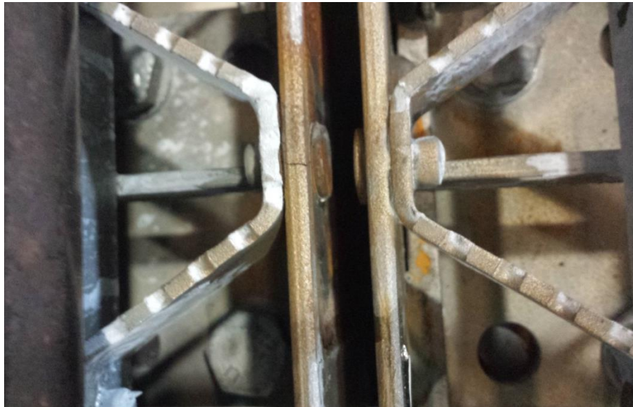
Figure 5.2 - Tension crack developed at edge of panel during Test 6
