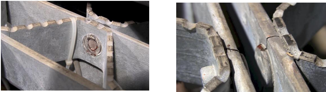
Figure 5.13 – Fatigue failure of components of the 37R5 L-series at 2 million cycles
