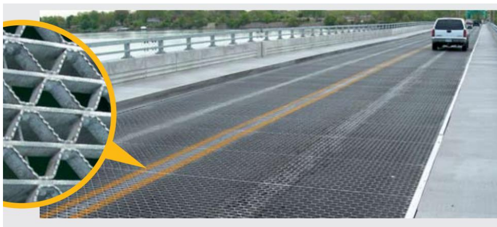
Figure 1.4 - Grosse Ile Bridge, Heavy Duty Riveted Grating installed in 2007
