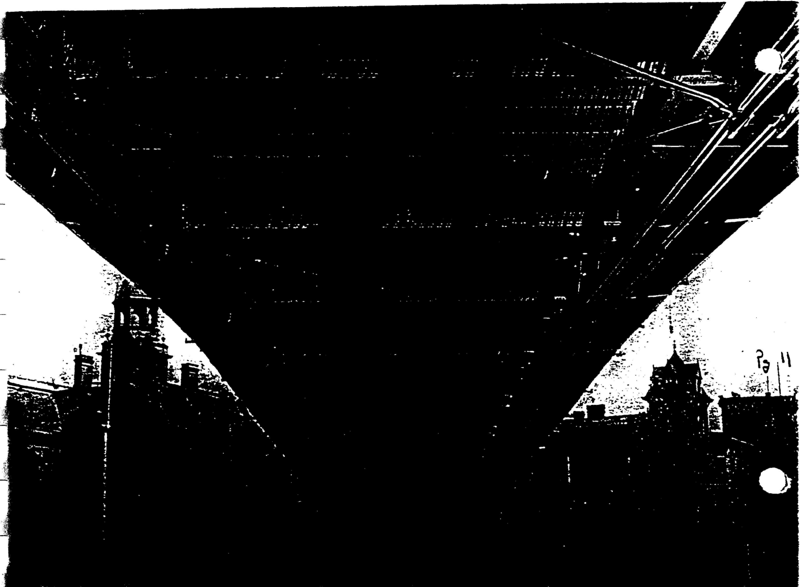
Reflooring Charleroi-Monessen Bridge, Charleroi, Pa., on which a total of 33,862 sq. ft. of 5" I-Beam-Lok Open Floor were used on the main spans and West approach viaduct St. Clair Street Bridge, Frankfort, Ky., for the Commonwealth of Kentucky, Department of Highways. Refloored with 9,720 sq. ft. of 5" I-Beam-Lok Open Floor
