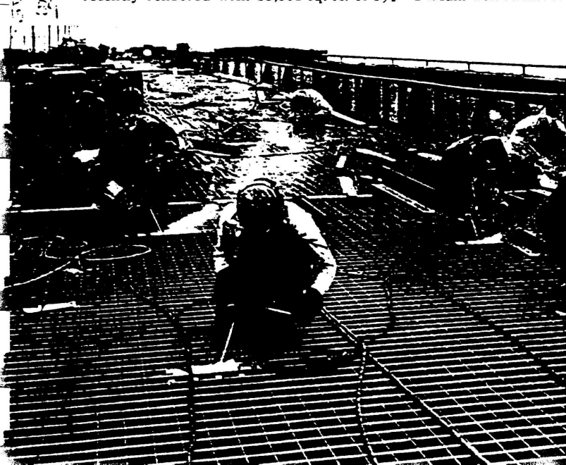
Doremus Avenue Bridge, spanning railroad tracks in Newark, N. J., recently refloored with 33,588 sq. ft. of 3½" I-Beam-Lok Armored
