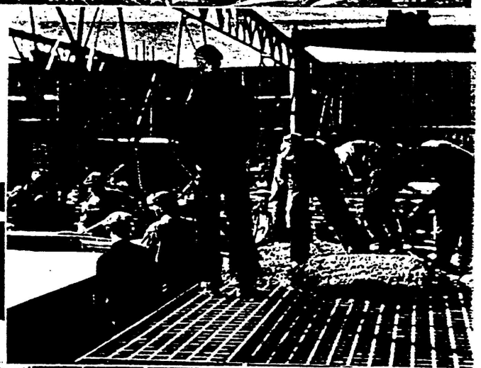
Pouring and finishing the concrete filled I-Beam-Lok panels
