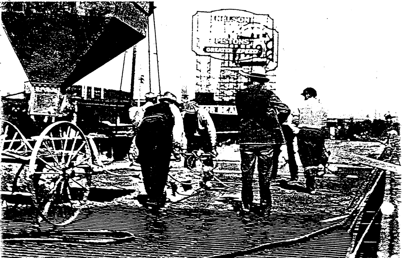
East Grand Boulevard Viaduct, Detroit, Michigan. Pouring, vibrating and finishing concrete
