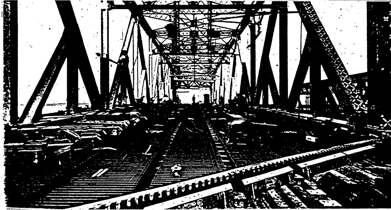
Torrence Avenue Vertical Lift Bridge, Chicago, Ill. Designed by the City of Chicago, Department of Public Works, Bureau of Engineering, Division of Bridges. Required 11,385 sq. ft. 3\frac{1}{2} " I-Beam- Lok Armored Floor
