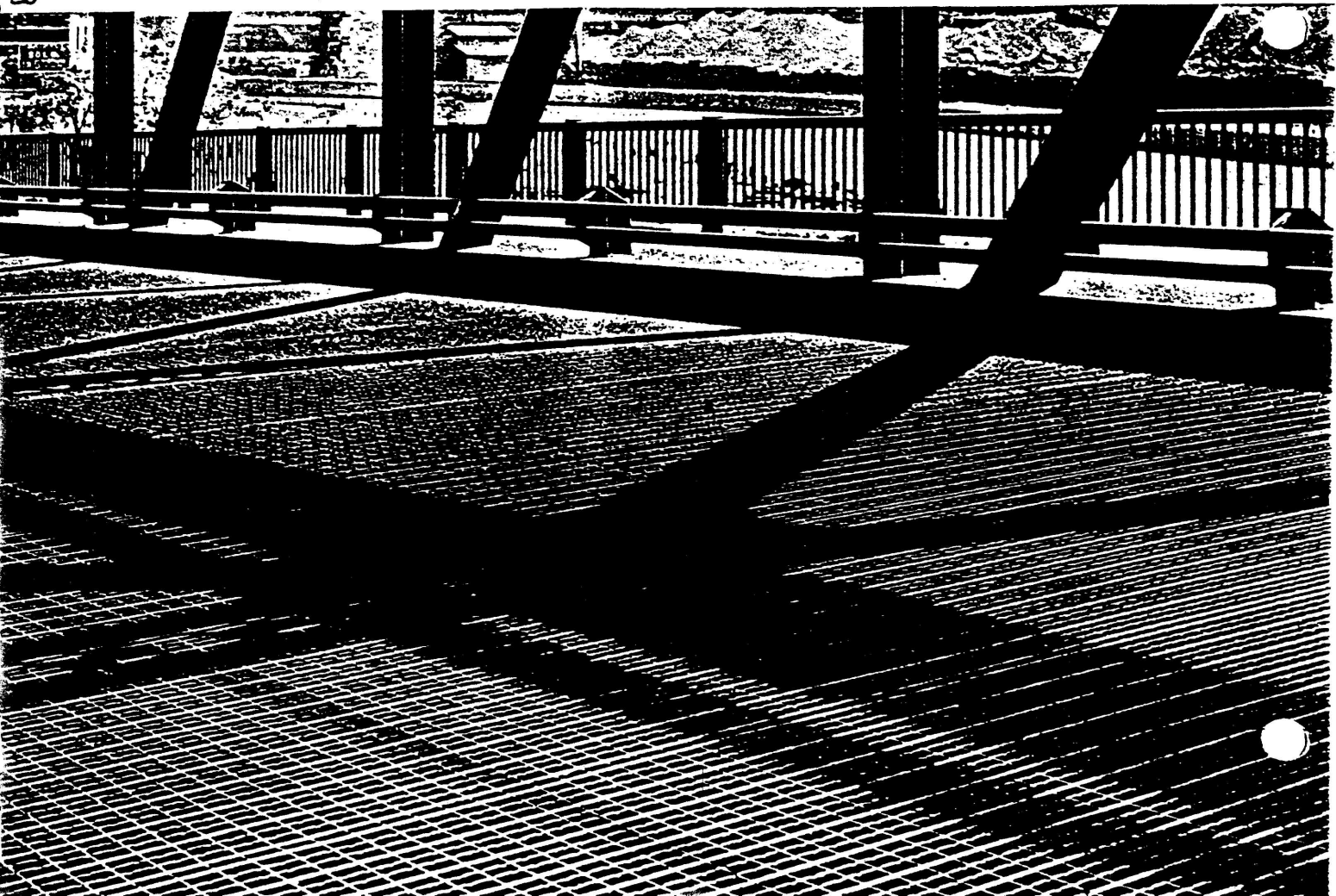
Northwest 27th Avenue Bridge over the Miami Canal, Miami, Florida. Designed by Harrington and Cortelyou, Consulting Engineers. Bridge required 6,300 sq. ft. 5" I-Beam-Lok Open Floor
