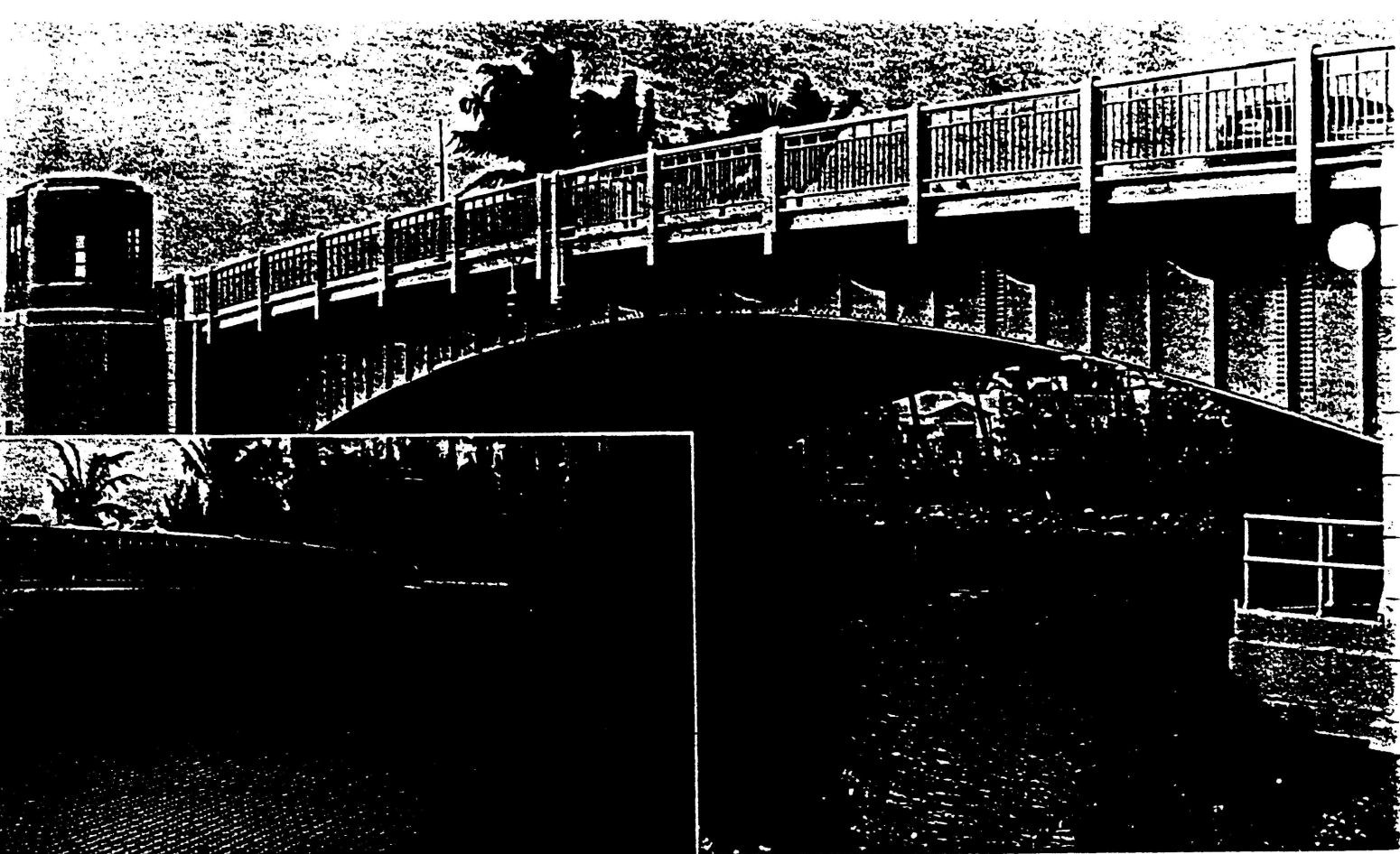
Northwest 27th Avenue Bridge over the Miami Canal, Miami, Florida. Designed by Harrington and Cortelyou, Consulting Engineers. Bridge required 6,300 sq. ft. 5" I-Beam-Lok Open Floor
