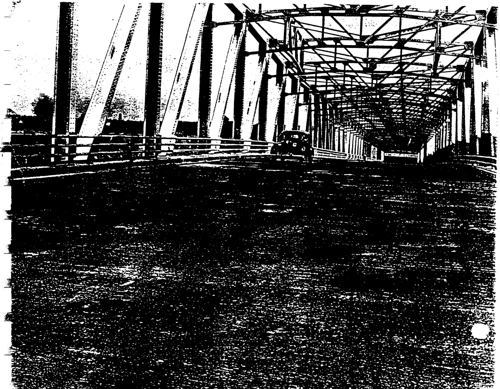
Two views of the East 21st Street Bridge, Lorain, Ohio. Wilbur J. Watson, Consulting Engineer. 72,000 sq. ft. of 4 \frac{1}{4} " I-Beam-Lok Armored Floor were used
