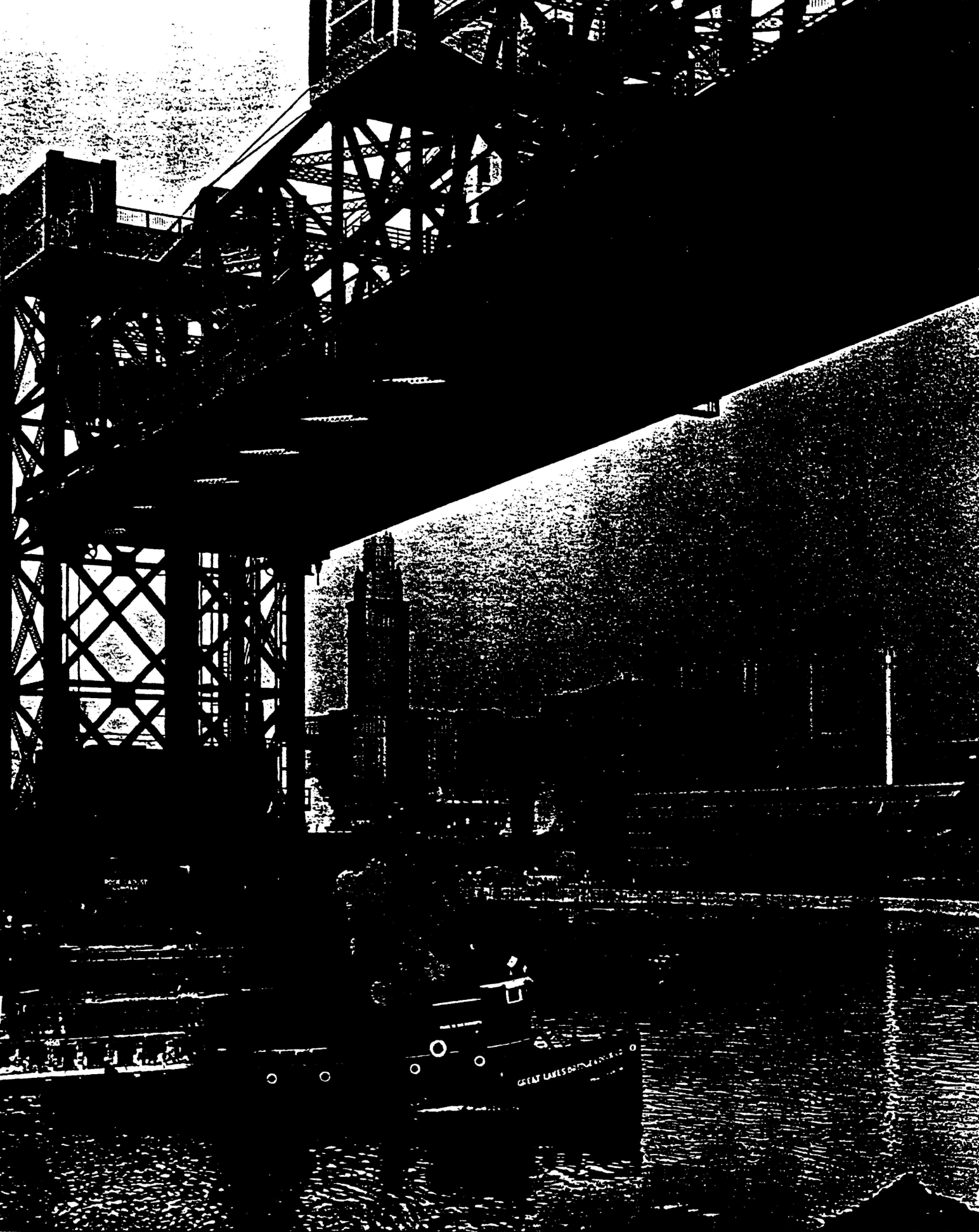
10,300 sq. ft. of U-S-S I-Beam-Lok Open Floor are used on the Roadway of this Columbus Road Bridge; 4,700 sq. ft. of Concrete filled 4\frac{1}{4} " I-Beam-Lok were used on the approaches and towers
