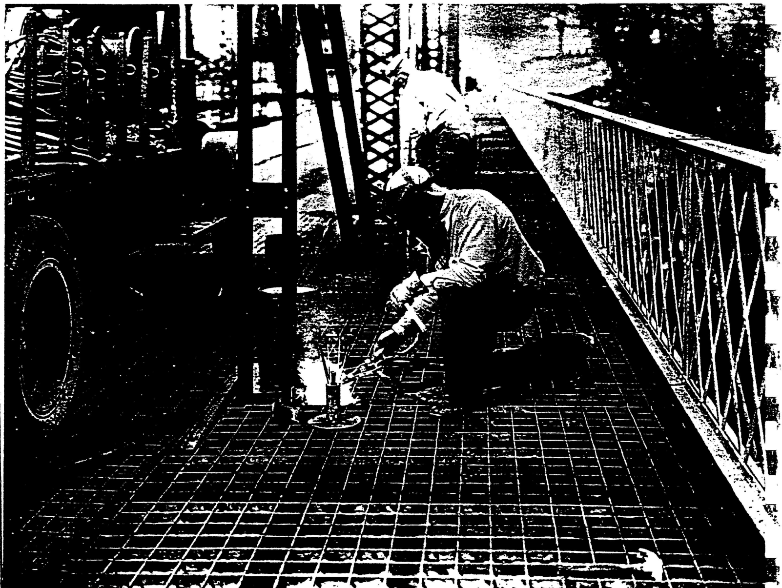
Field welding 2" T-Tri-Lok sidewalk unit to the supporting steel
