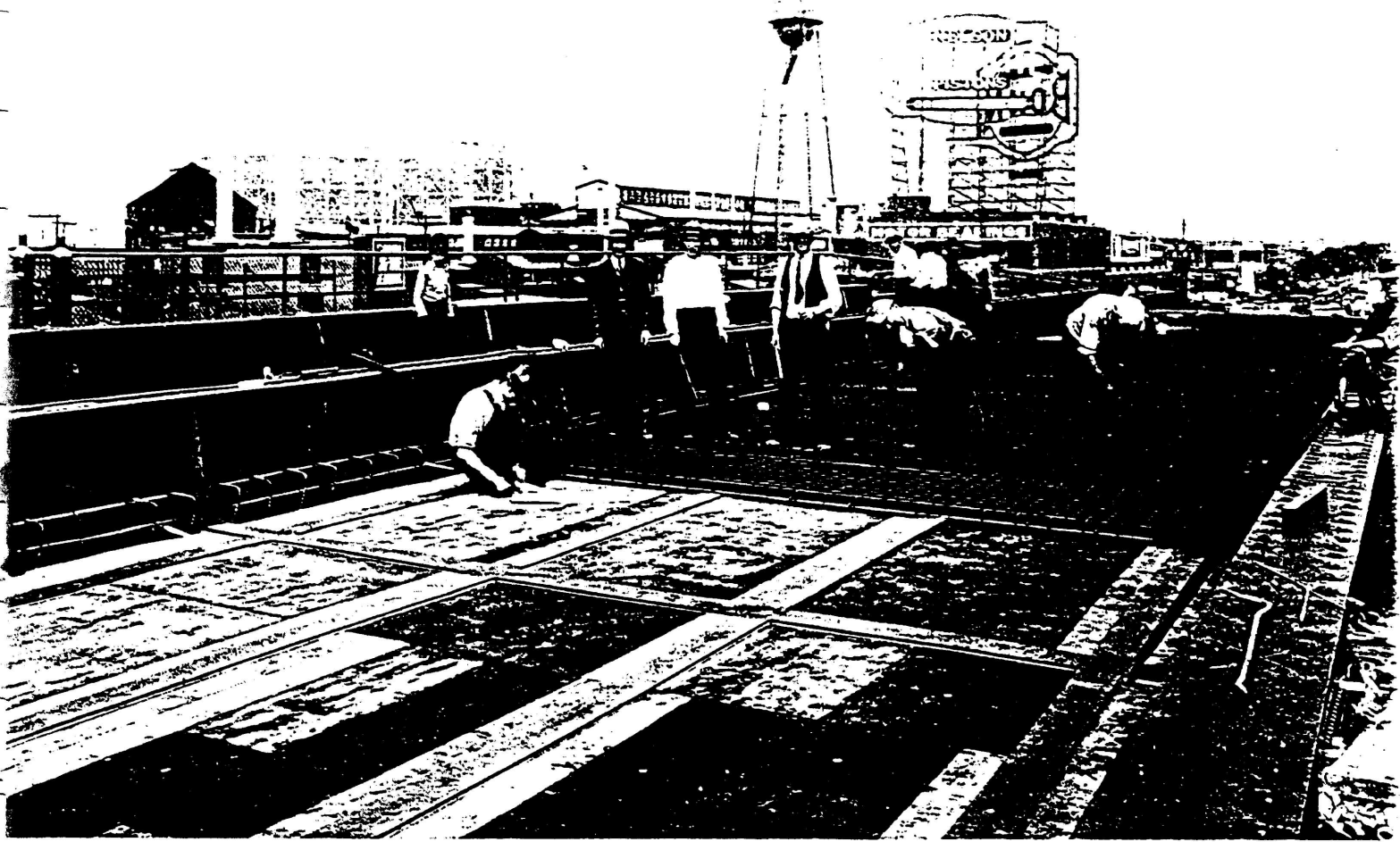
East Grand Boulevard Viaduct, Detroit, Michigan. Steel form strips omitted over rail-road tracks. Wood form placed 3' below I-Beam-Lok steel to secure concrete cover
