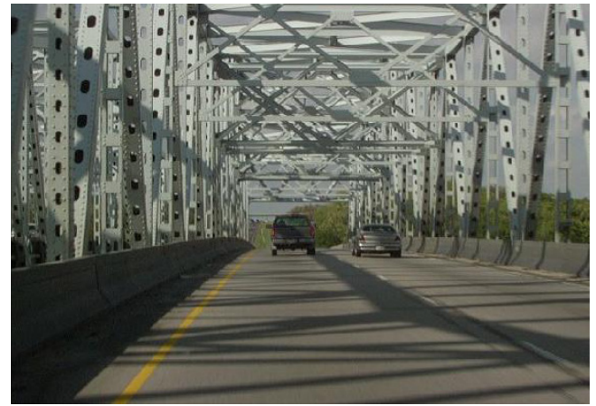
Interstate 55 Bridge Full-Depth Grid Deck
